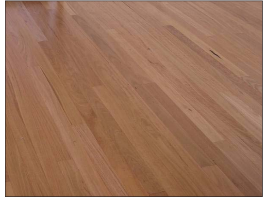
A select grade Blackbutt floor where the backsawn gum vein toward the top right exceeds grade limits but is acceptable within the floor.
